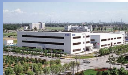
SMC (China) Co., Ltd. Total Land Area: 172,556 m 2 Floor Space: 85,819 m 2
