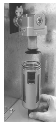
Pull down the case assembly slowly
